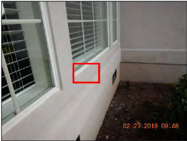
Damage / visible mesh at EIFS window trim detail. Repair all damage.
