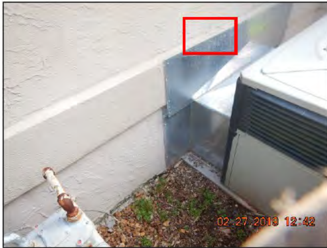
(1) Caulk failing at HVAC ductwork shroud. Recommend repair / caulk as needed.
