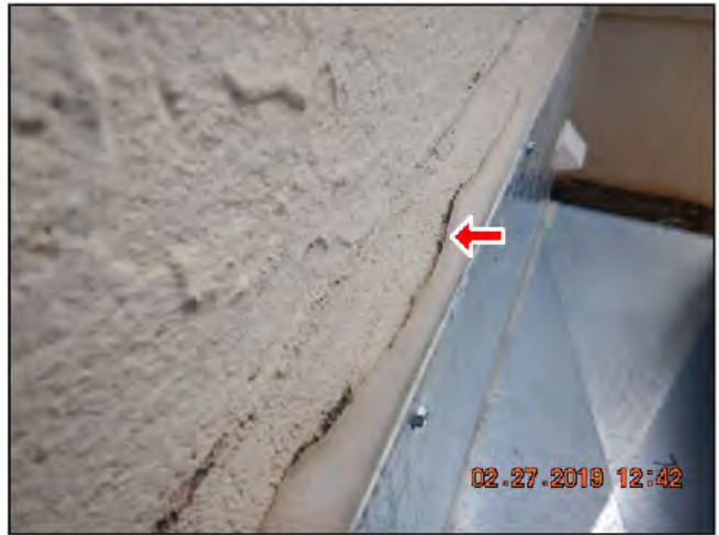
(1) Caulk failing at HVAC ductwork shroud. Recommend repair / caulk as needed.
