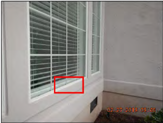
Caulking failing at window. Typical at most window. Recommend repair / caulk as needed.
