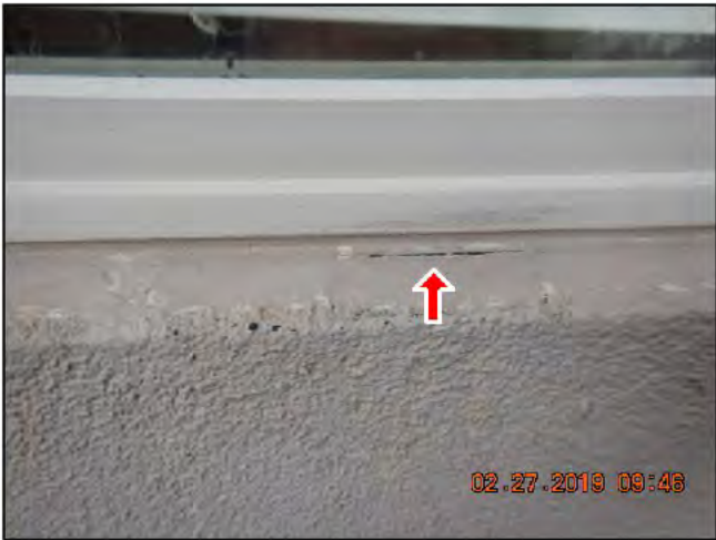
Caulking failing at window. Typical at most window. Recommend repair / caulk as needed.
